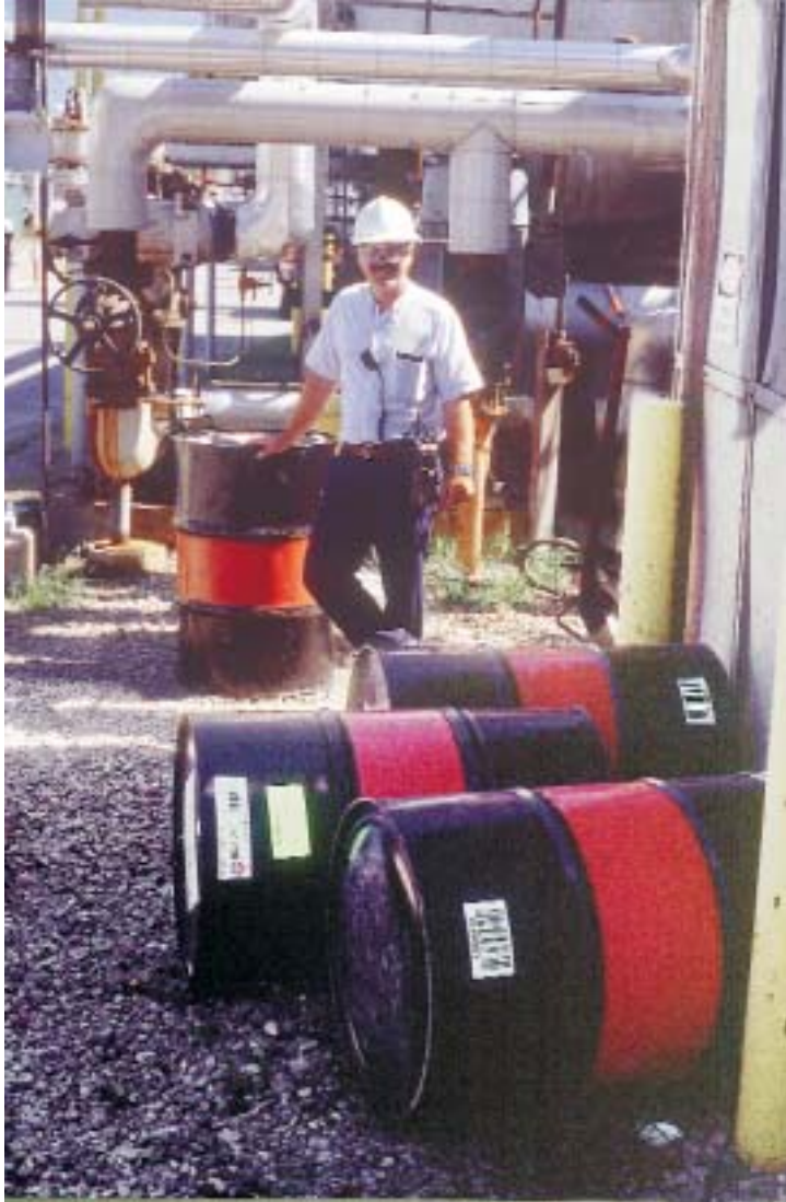
■ Gary Papalia, Assistant Zone Maintenance Superintendent for United Refining Company, stands behind what used to be a day's supply of seal oil. Now, with Kaydon seals, one barrel lasts 5 months.
